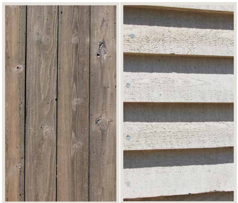
Horizontal and vertical natural wood siding in lapped, butt, and tongue and groove configurations are encouraged.
